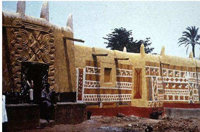
Figure 3: Decorated house facade in Zaria, Nigeria: painted facade and mud relief. Source: Tetteh, (2010) http://pitt.edu/tokerism
