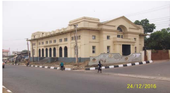
Figure 6b: Pictorial view of the Centenary Hall Ake, Abeokuta-Nigeria built in 1930 (The building typifies the obliteration of traditional architectural styles by European influence). Source: Authors, (2016.)
